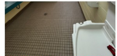
EXISTING WOMEN'S RESTROOM
