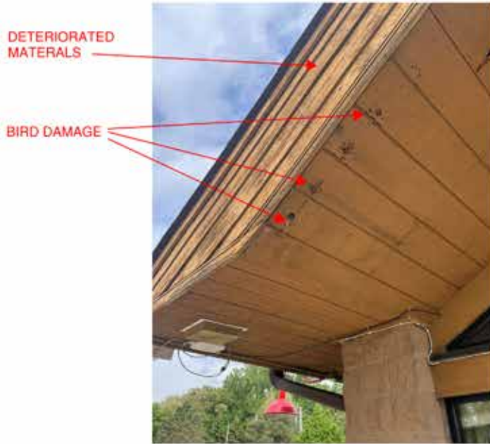
SOUTHEAST CORNER OF EAVE
