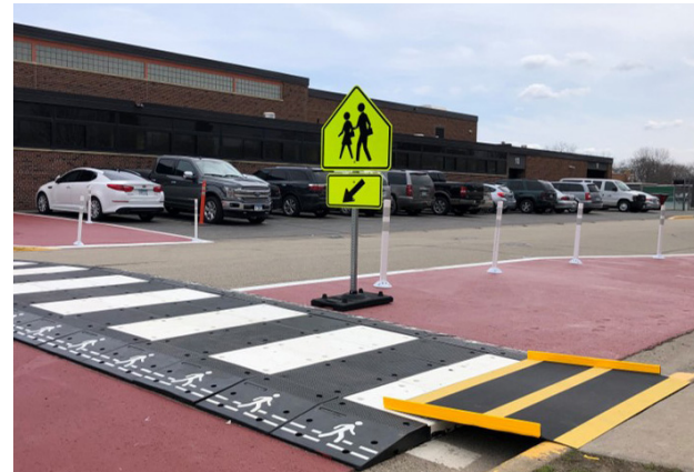
This raised crosswalk connects to a school entrance and slows traffic on the adjacent road.
